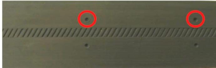
Make sure that there is a screw about 1 inch (2½ cm) or closer to each end – if necessary, by adding a screw or two.
