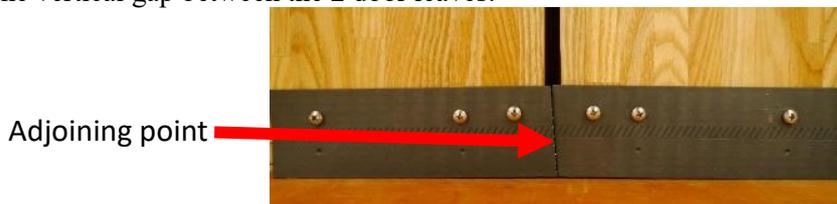
Do not make the 2 pieces overlap. It is OK if there is a very small gap of up to 1/16 inch (1.5 mm) between the 2 pieces of door sweep.
