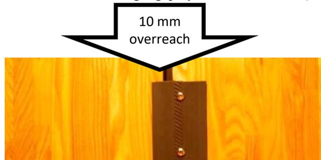
**G.** The screws should as a main rule be placed around the middle of the proofing strip and not as indicated by the screw hole markings. E.g. if the astragal gap is 6/16 inch (10 mm) broad it should be mounted like this:
