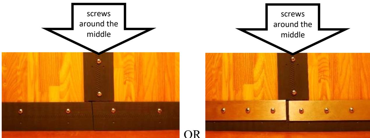
**H.** Fasten the uppermost screw first. Thereafter, continue downwards placing a screw for each around 4 inches (10 cm) until you reach the bottom end of the proofing strip.
